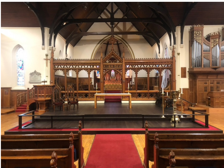
Photo 2 - New sanctuary altar platform after construction (note extra height and removeable handrails)
